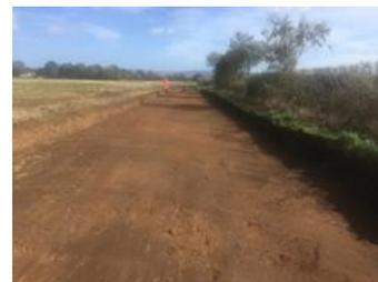
**Coming up...**Over the next two to three weeks work will be completed on the carrier drains, the levels will be finished off to prepare the land for the pitches within the perimeter of the fitness track and the area to the rear of the skate park will be regraded (23 – 26 October).
